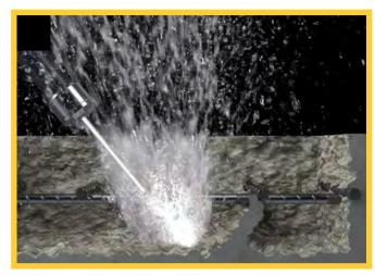
By exposing the concrete to the water jet for a certain time you reach the desired depth.
