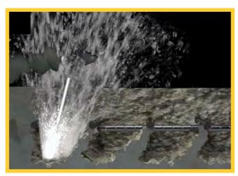
By changing the angle of the lance the remaining material under the rebar (the shadows) will be removed.
