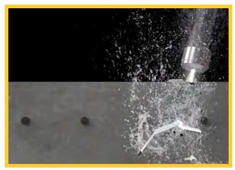
The water jet penetrates existing cavities and cracks.
