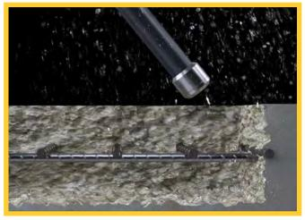
The remaining area consists of structurally sound concrete and is now prepared for the application of a new layer.
