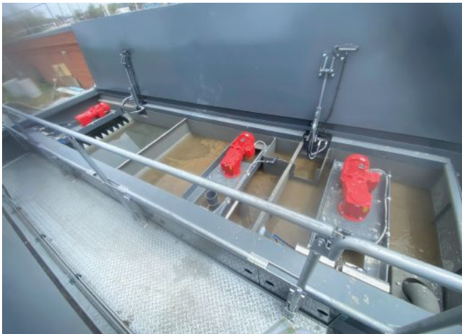
Fig. 7: Hydrodemolition wastewater treatment process.
