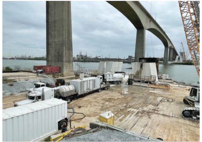
Fig. 6: Staged water supply and recycling equipment during hydrodemolition.
