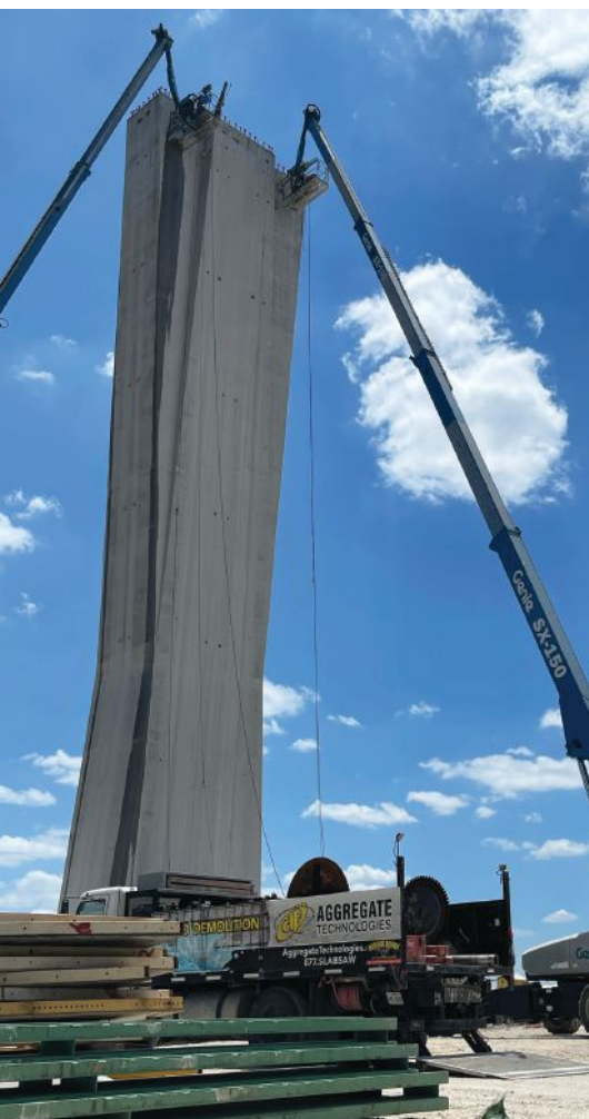
Fig. 3: Initial stages of pylon removal.
