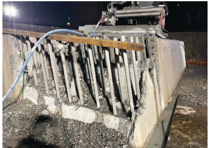
Fig. 8: Active hydrodemolition on elevation.
