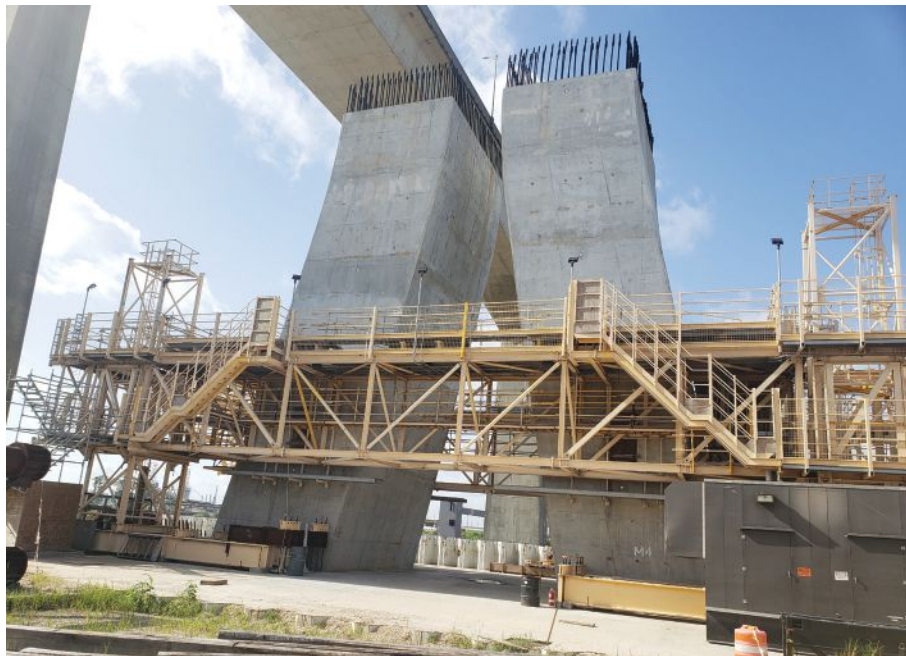
Fig. 2: Two of four pylons wrapped with scaffolding.
