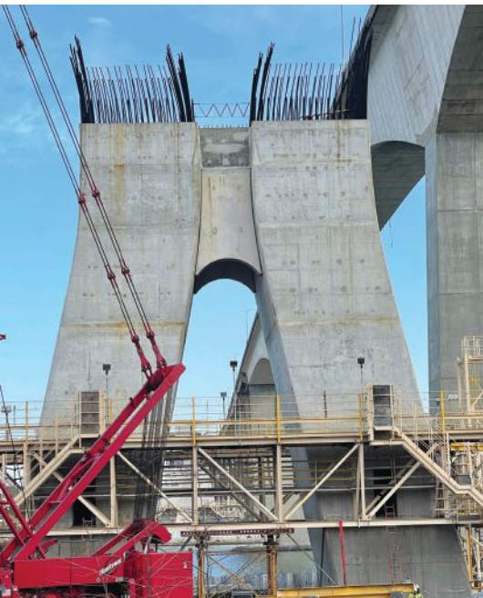
Fig. 1: The stage is set for the top-down demolition with rebar retention.
