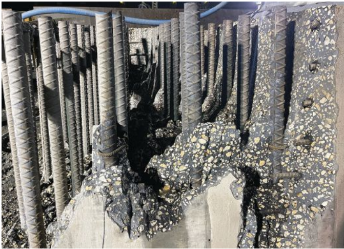
Fig. 5: Close-up of concrete being removed from rebar during hydrodemolition.
