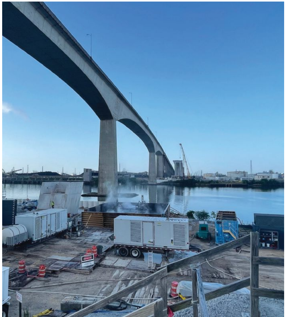
Fig. 10: Final stages of pylon removal.
