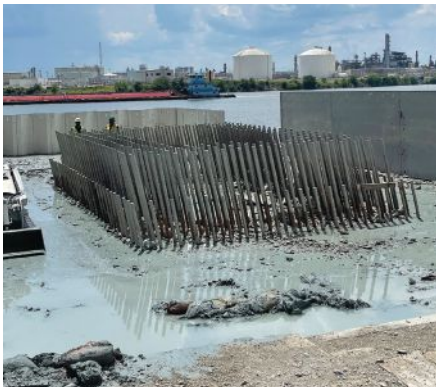
Fig. 9: Completed removal of pylon with exposed rebar.
